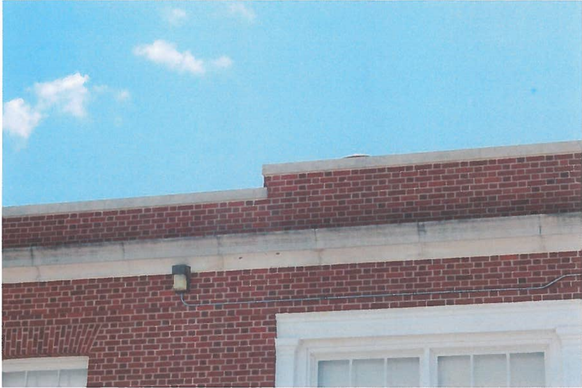
Stone parapet cap and cornice at east side of building.
