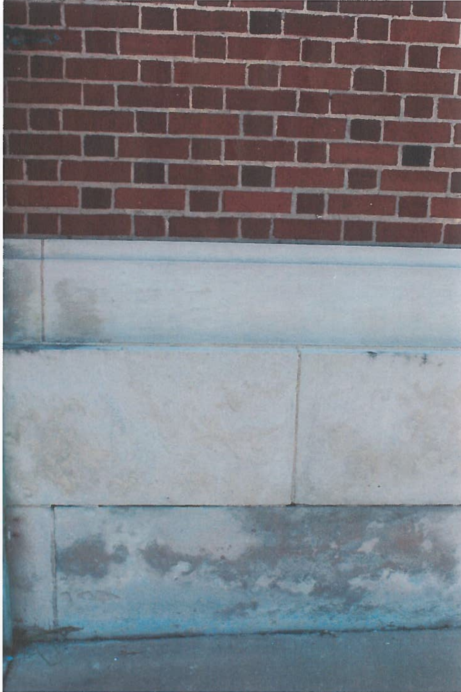
View of typical stone base at mechanical yard.
